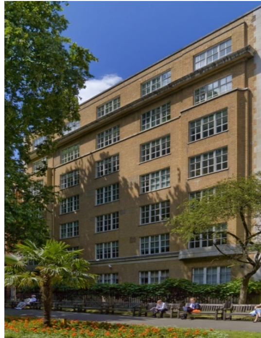
<Back of building>
